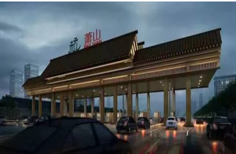
Hangzhou Xiaoshan Toll Station
