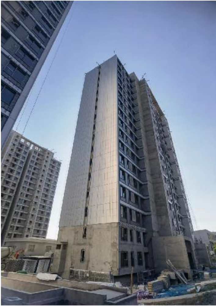
Zhongtong, Gaoyuan Construction
